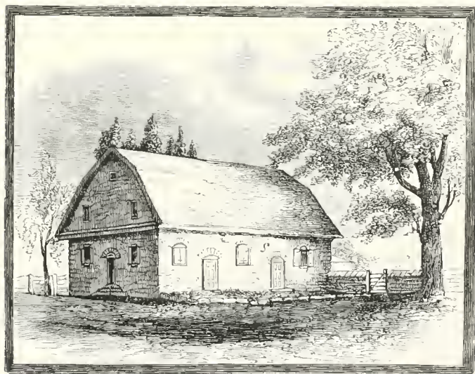
SPRINGFIELD MEETING HOUSE, DELAWARE COUNTY BUILT 1738. TAKEN DOWN, 1850
